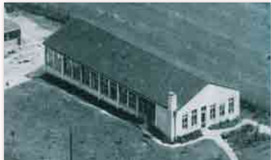
New building I: Operations boom just five years after it was founded the company moves into a new building in Marbach, where it is still located today.
